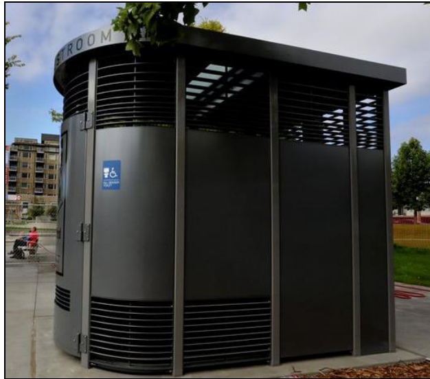
Portland Loo installation in Seattle, WA.
